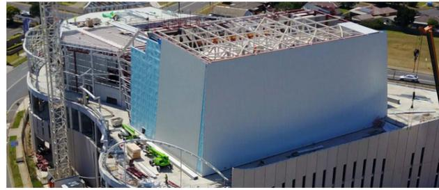
The external Colorbond® walls behind the theatre space were lined with Sisalation® Metal Roof 453 Heavy Duty roof sarking and FI48 75mm Rigid glasswool insulation (Wall Schematic).
