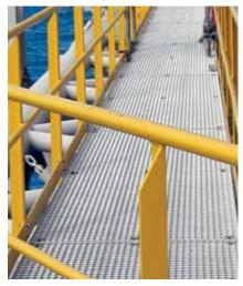
Weldlok® aluminium grating at Abbot Point Coal Terminal, Qld
