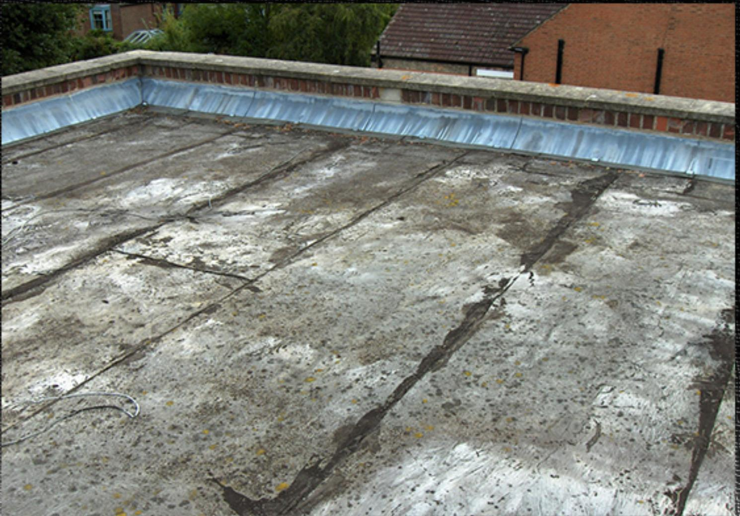
The refurbishment of a failed flat roof is the most common waterproofing problem that the building industry is coming across. Taking all the variables into consideration when specifying a waterproofing solution is not an easy process.
