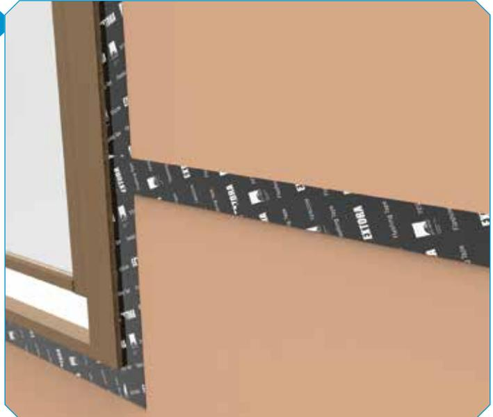
TESCON EXTORA® is a pressure sensitive tape that requires sufficient pressure to activate the adhesive. Always ensure you use a PRESSFIX® (or a 100mm joint knife or similar if a PRESSFIX® is not available) when installing TESCON EXTORA® to activate the adhesive and achieve a permanent bond. Please be aware, once the adhesive has been activated, the tape cannot be removed.
