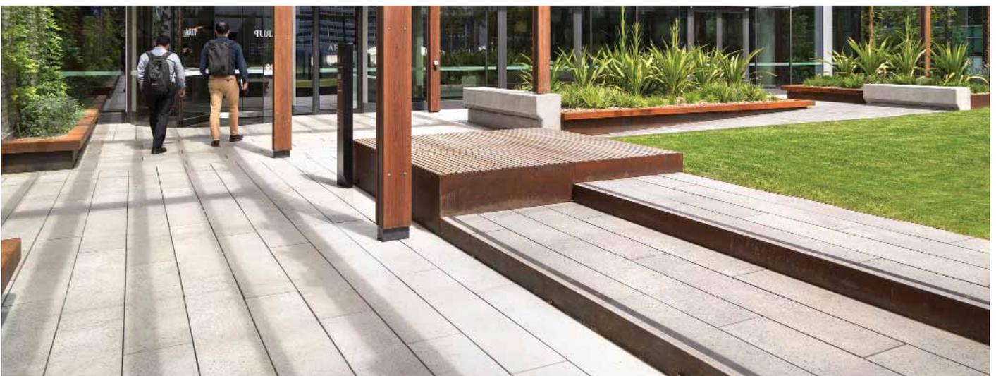
Exposed aggregate paving planks at Melbourne Quarter Skypark. Design: OCULUS & Aspect Studios for Lendlease
