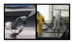
Polyurea applied to concrete deck plate
