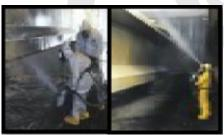
Polyurea being applied to concrete girder
